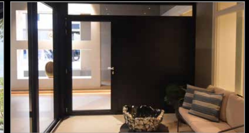
\ Aluminum wall, glass door and glass panel
